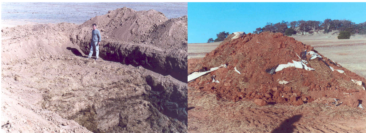
Figure 1. 0.8 m soil removed from stack top Figure 2. Soil contaminated with plastic
