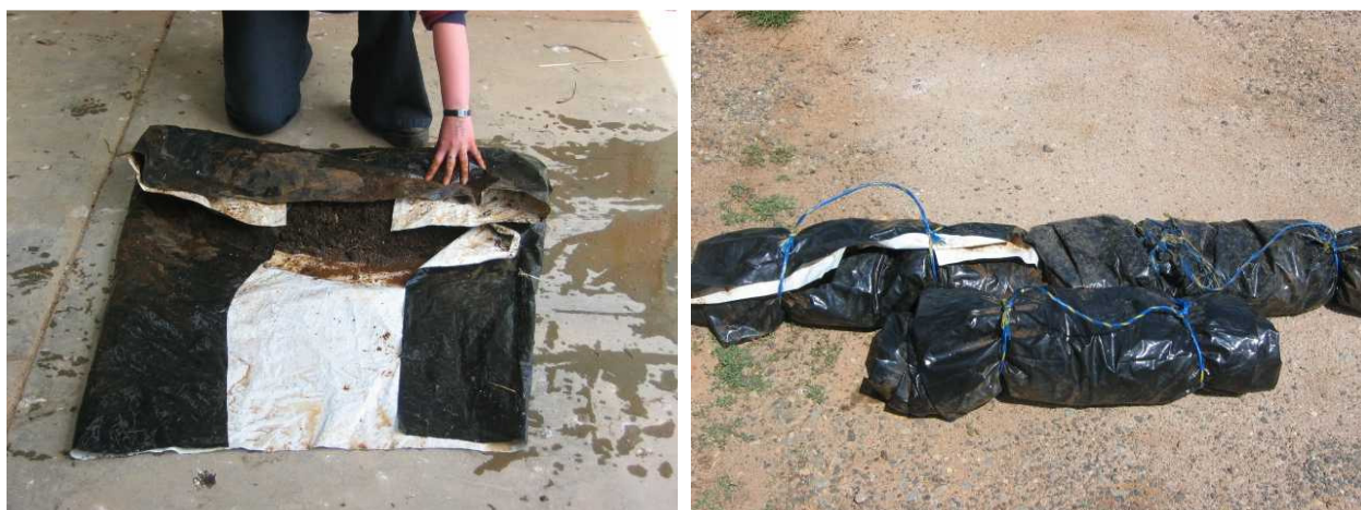
Figure 1a & b. “Sausages” made from old plastic, gravel and large square bale hay twine
