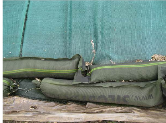
Figure 2b. Gravel socks overlapped
