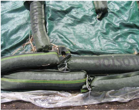
Figure 2. Sausage filled with gravel, made from waste plastic sheet
