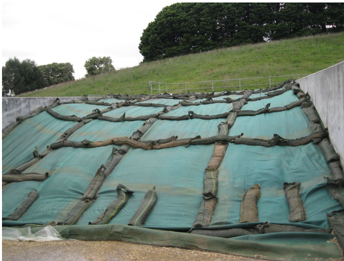
Figure 3. Gravel socks sealing stack front, edges and surface
