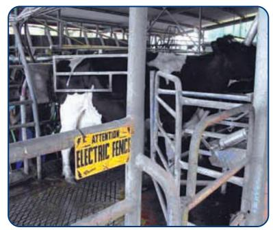
Figure 4.13: Electric fence units and wires that contact dairy pipework are a common source of stray voltage.
