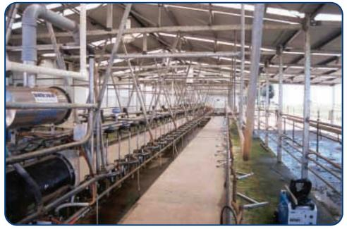
Figure 4.10: Good open dairy design with straight in, straight out cow movement through the dairy. Source: National Milk Harvesting Centre.
