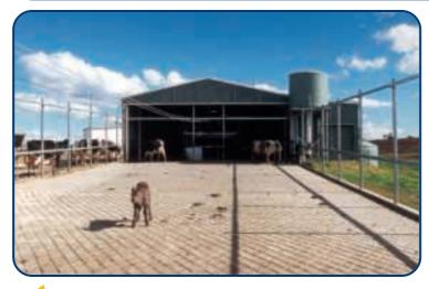
Figure 4.4: Single slope yard with grooving all running down slope. Source: National Milk Harvesting Centre.
