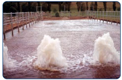
Figure 6.8: Flood wash system with sub surface riser. Source: National Milk Harvesting Centre.
