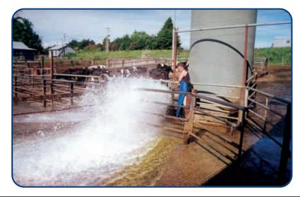
Figure 6.7: Flood wash option – large water tank in yard.
