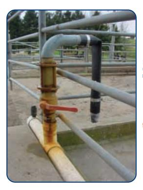
Figure 6.5: Hydrants with an industrial swivel are safer to use. Source: National Milk Harvesting Centre.
