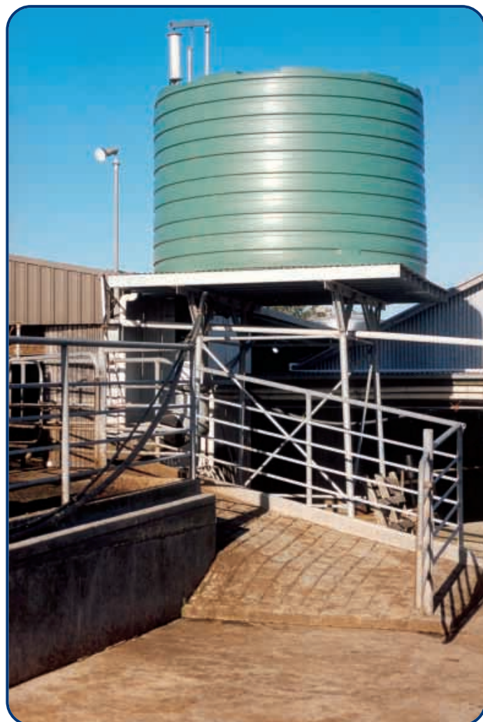
This photo shows the floodwash tank.
