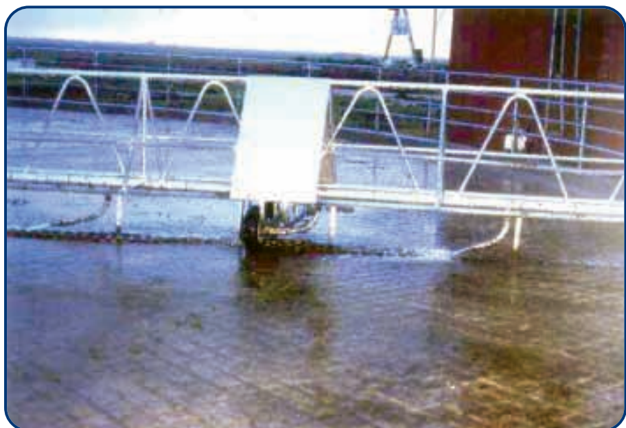
This picture shows the backing gate with chains and water outlets on David and Cathy's yard.
