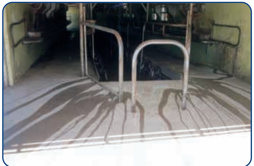
This photo shows the dribble bar at the entrance to the dairy before any cows have entered the dairy.
