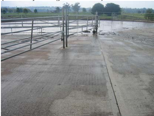
3. Holding yards (from dairy looking towards rear)
